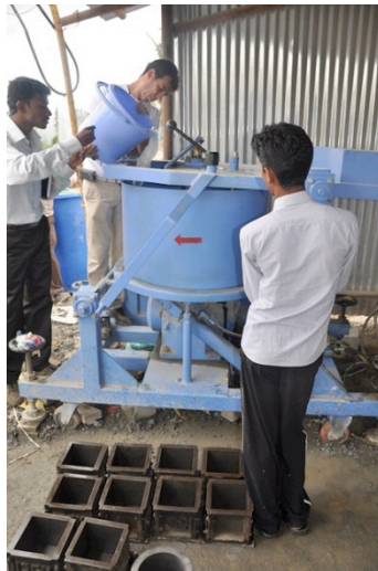
PHOTO 9. Adding water with MAXEH to dry soil-cement mixture.
