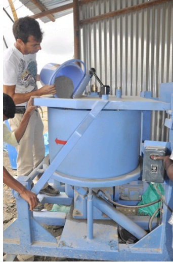
PHOTO 8. Pouring cement into dry soil.
